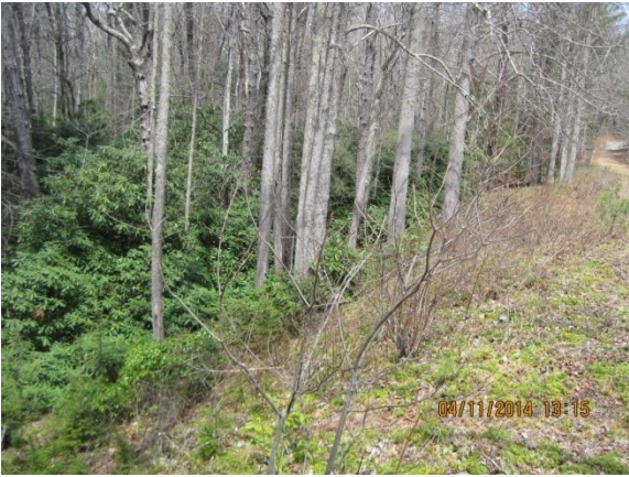
Trees and thick underbrush on dam
