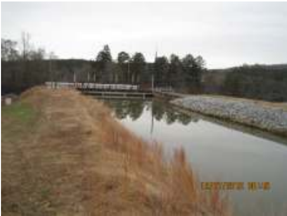
channel leading to power house
