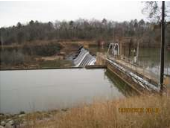
channel leading to power house
