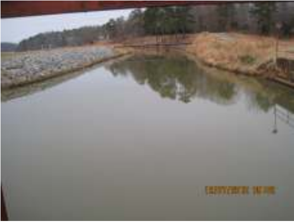
channel leading to power house
