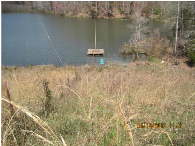
Upstream slope of dam
