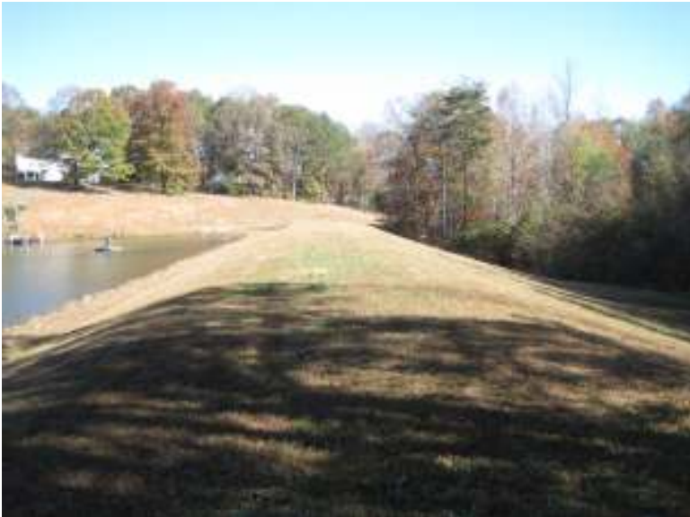
Crest of dam
