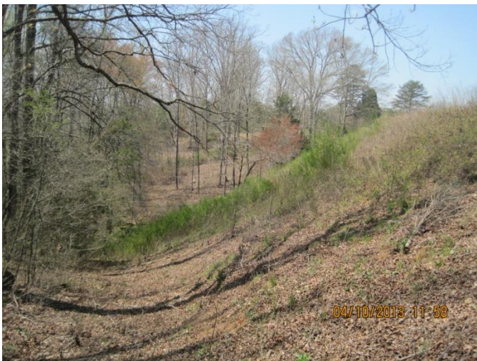
Downstream slope of dam
