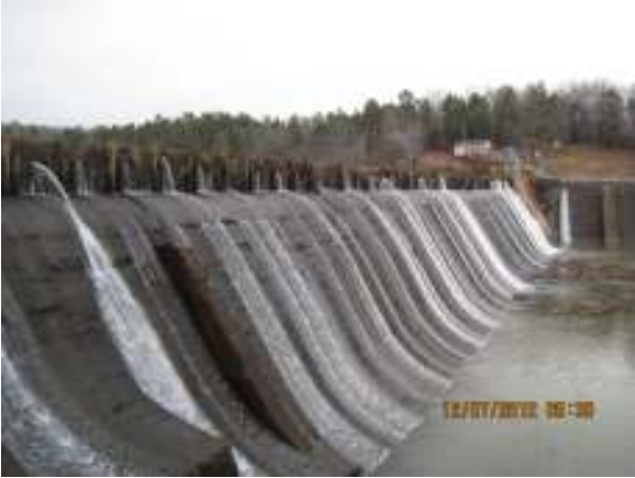
flashboards and downstream slope of dam
