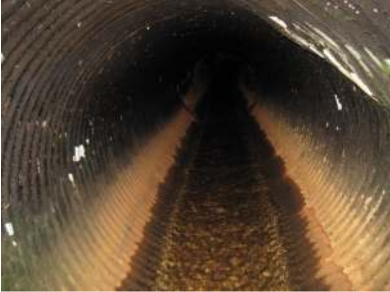
Inside of discharge pipe
