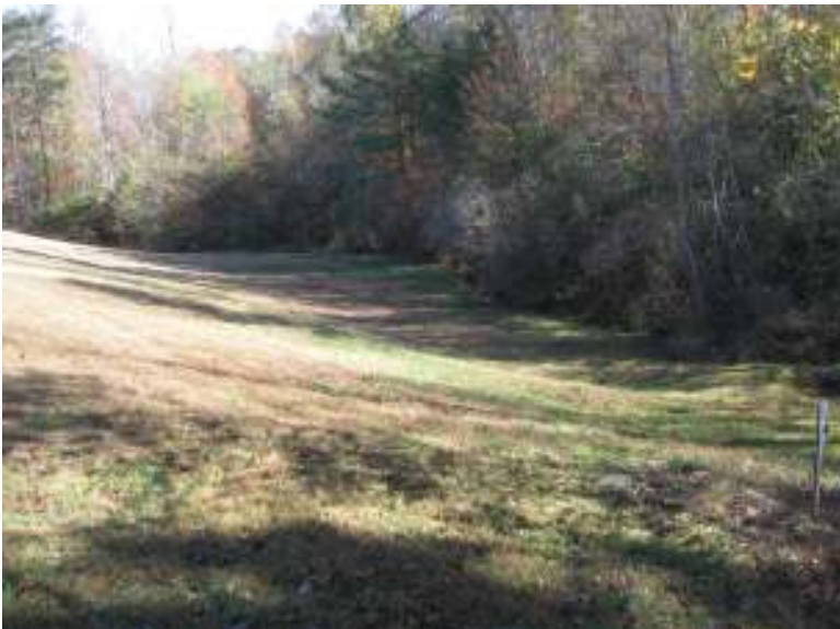
Down stream slope of dam
