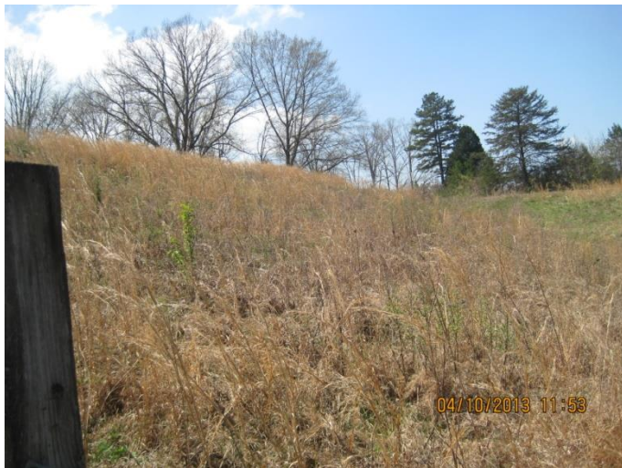
Upstream slope of dam
