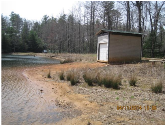
Boat shed constructed on dam
