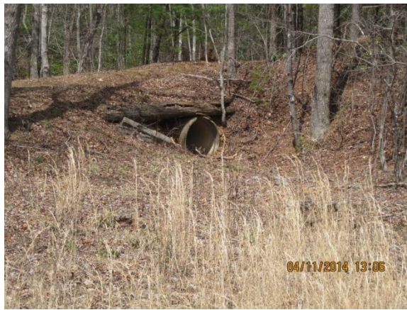
Large concrete pipe for emergency spillway
