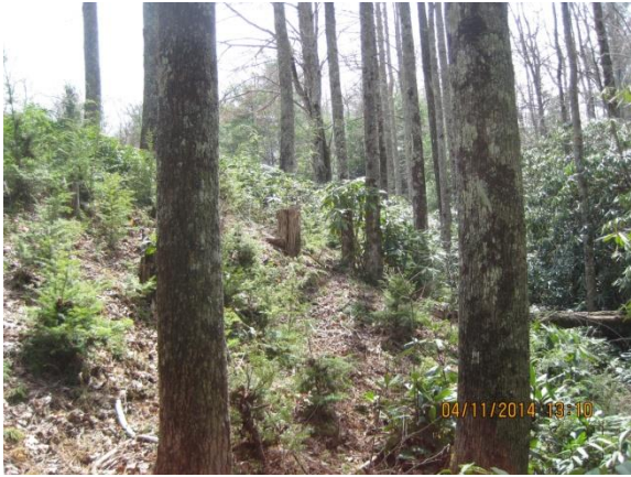
Large trees on dam
