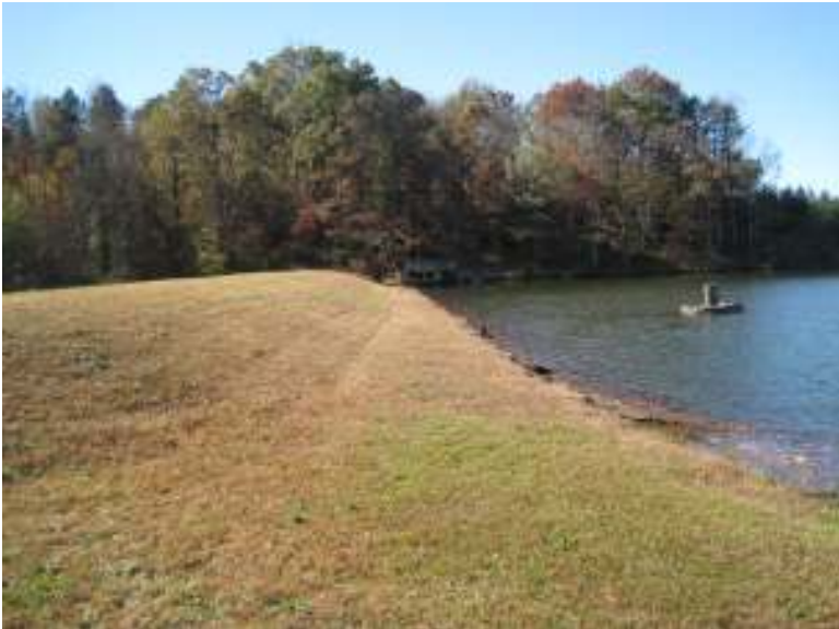
Upstream slope of dam
