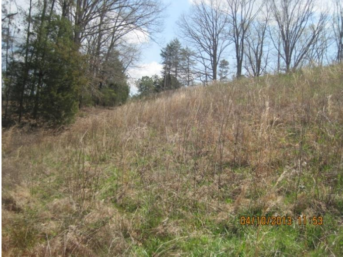
Upstream slope of dam
