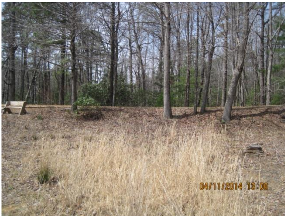
Trees on dam
